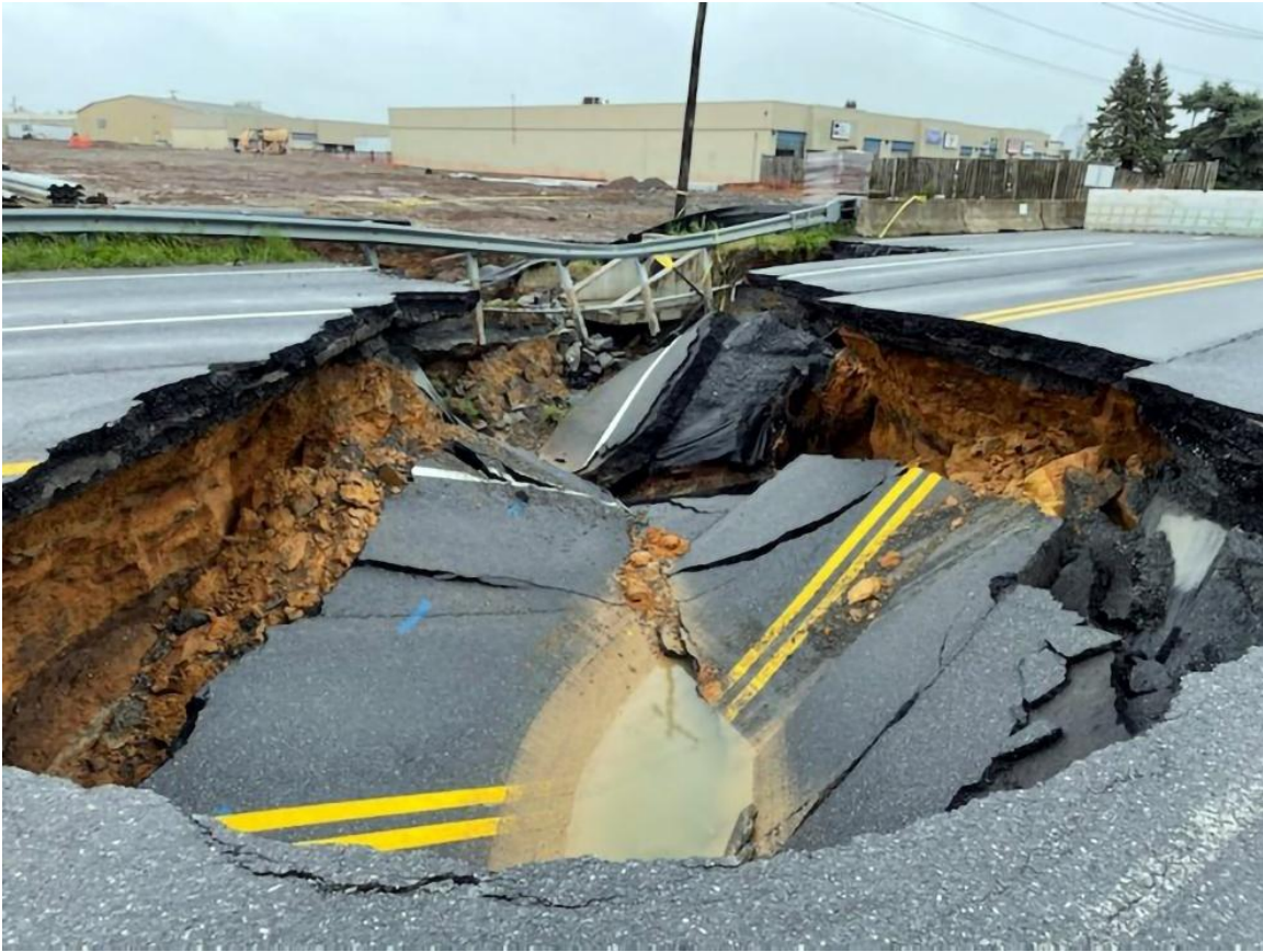
Figure 28 - Sinkhole formed in a street in Frederick, Maryland, USA, on May 7, 2022. Dye and flush water were introduced into this collapse for a successful trace.
